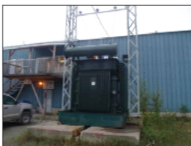
(a) 2000KVa transformer, 3 Phase 600V from 24Kv primary
